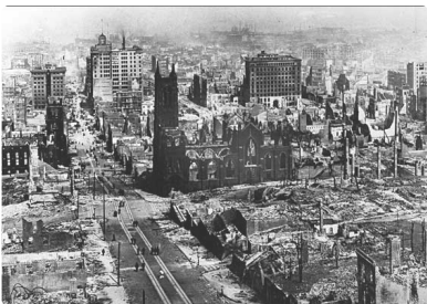
In the San Francisco quake of 1906. Broken gas pipes ignited fires
