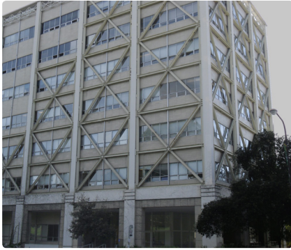
California is an area of strong earthquakes. Here: a house strengthened
